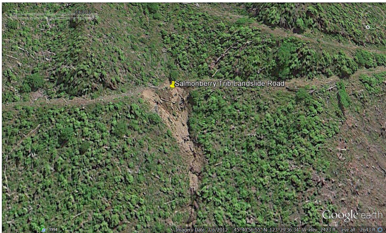
Road-related landslide in the Salmonberry Watershed.
