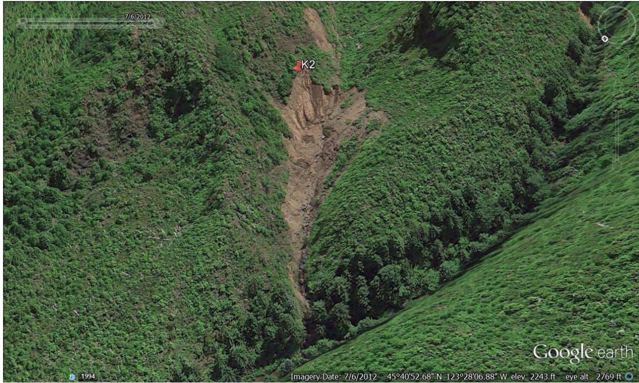
Landslide into Kinney Creek, South Fork Salmonberry Salmon Anchor Habitat.
