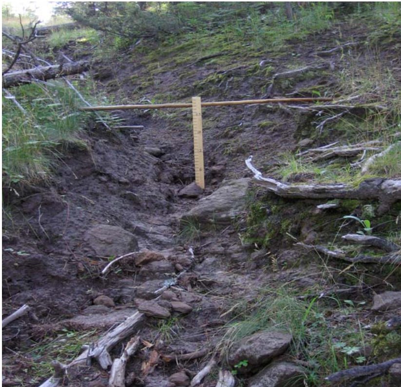
Severe erosion and downcutting on Cross-town trail caused by motorized use.
