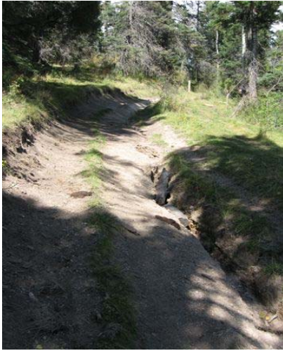
Severe Erosion on FR 282.
