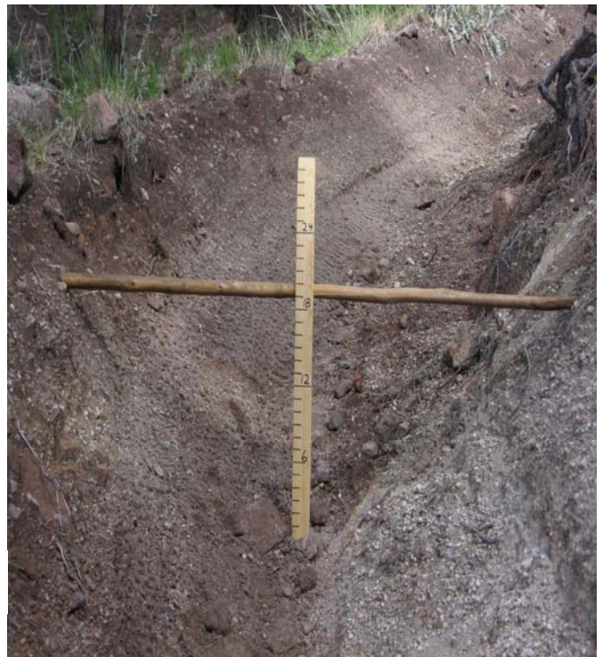
Severe soil erosion on FT 113 from motorized use.
