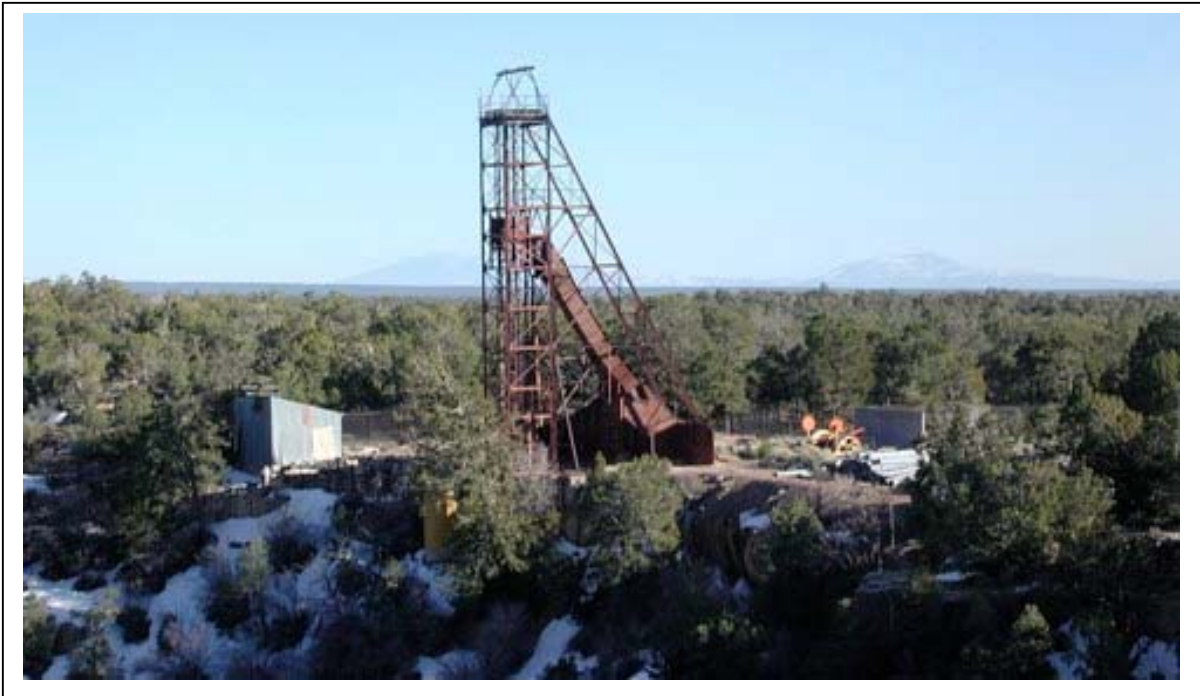
Figure 3. Orphan Mine headframe and mine yard, South Rim Grand Canyon National Park. Snow on slope melts, facilitating release of contaminants to Horn Creek below. (Photo by C. Shuey, 3-27-08)
