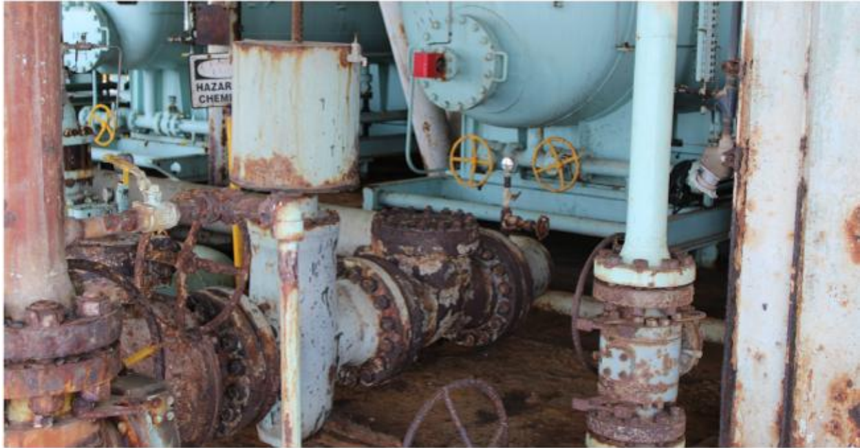
Figure 8. Corrosion on Platform Hogan, which has been due for decommissioning since 2020. 192
