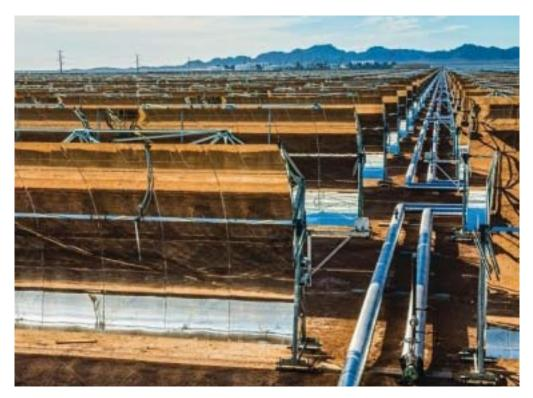
INTO THE HORIZON The Abengoa Solana concentrating solar power project began operating this year at Gila Bend, Ariz., generating 280 MW, using a system of parabolic troughs.
