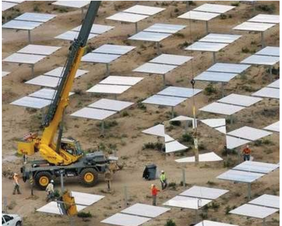
Workers install heliostats (software controlled directional mirrors) on the Ivanpah solar thermal power system in August. The Palen facility will use similar technology. / Jay Calderon, The Desert Sun
