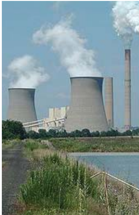
American Electric Power's coal-fired Gavin power plant on the Ohio River. Clouds of acid gases are emitted from the vertical column stacks, while the cooling towers emit water vapor. (Photo by Analogue Kid)
