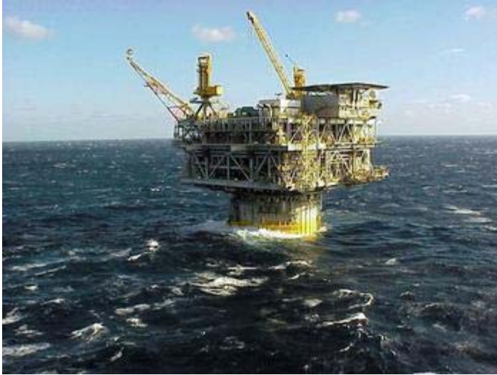
The Deep Draft Caisson Vessel built by Exxon Mobil for oil production in the Gulf of Mexico. At 75 stories tall and moored in 4,800 feet of water, this is the world's deepest drilling and production platform. May 26, 2010 (Photo courtesy U.S. Coast Guard)
